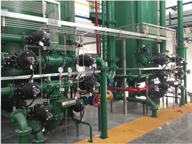
Boiled water system in coal power station
