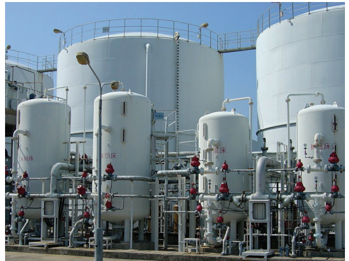
Desalted water in petro chemical plant
