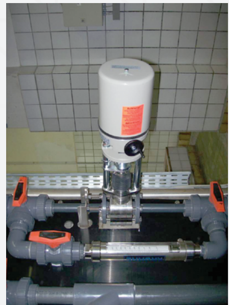
SSC Sliding disk valve with electric actuator in a water treatment plant
