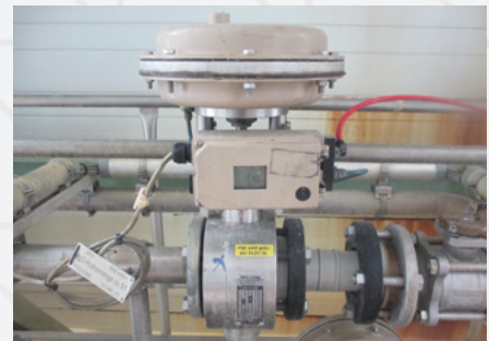
SSC Sliding disk valve with pneumatic SAMSON® actuator and positioner
