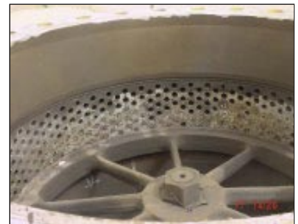
Pressure-balanced, axial flow valve This perforated trim design is not suitable for the existing process conditions.
