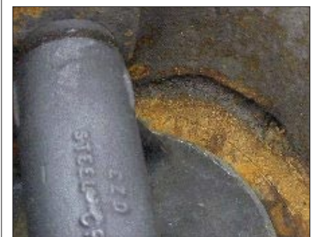
Fig. 31: Plant shutdown due to “quick and dirty” sizing with 8 inch rotary plug valve and too small DN.
